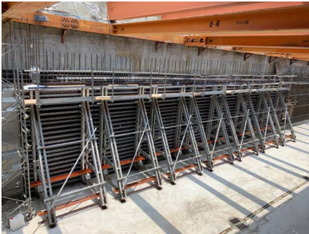
Kinmen Bridge - Pier Table (Box Girder H:7.5M) System Formwork & Access Tower
