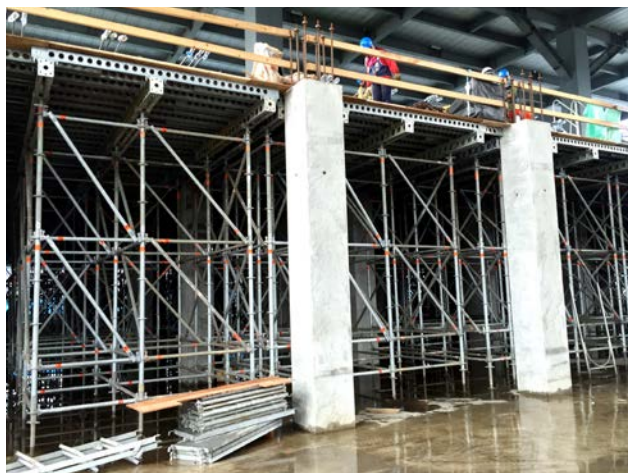
Taoyuan Longtan LY3 Factory Slab Formwork & Shoring
