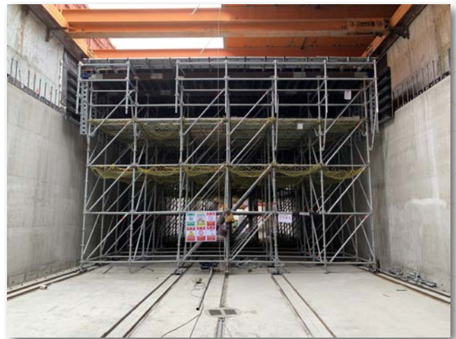
Cut and Cover Tunnel Slab System Formwork & Shoring
