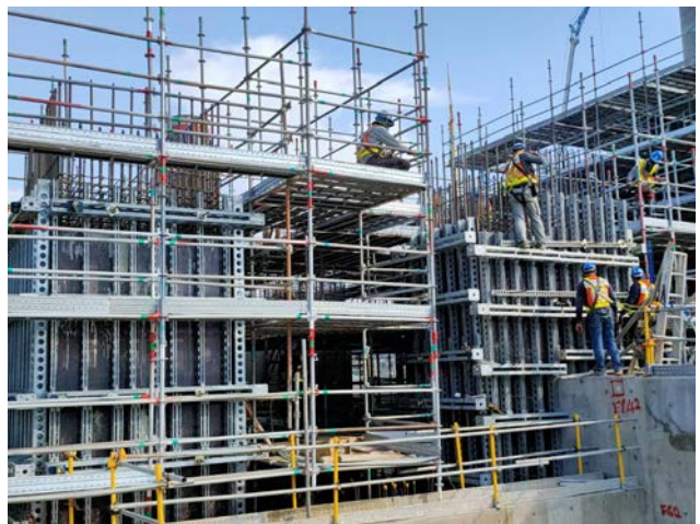
Datan Power Plant #7 STG Building 5.3M High Column Formwork
