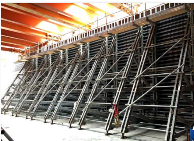
Tainan Underground Railway #C214 6.0M Single-Sided Wall Formwork
