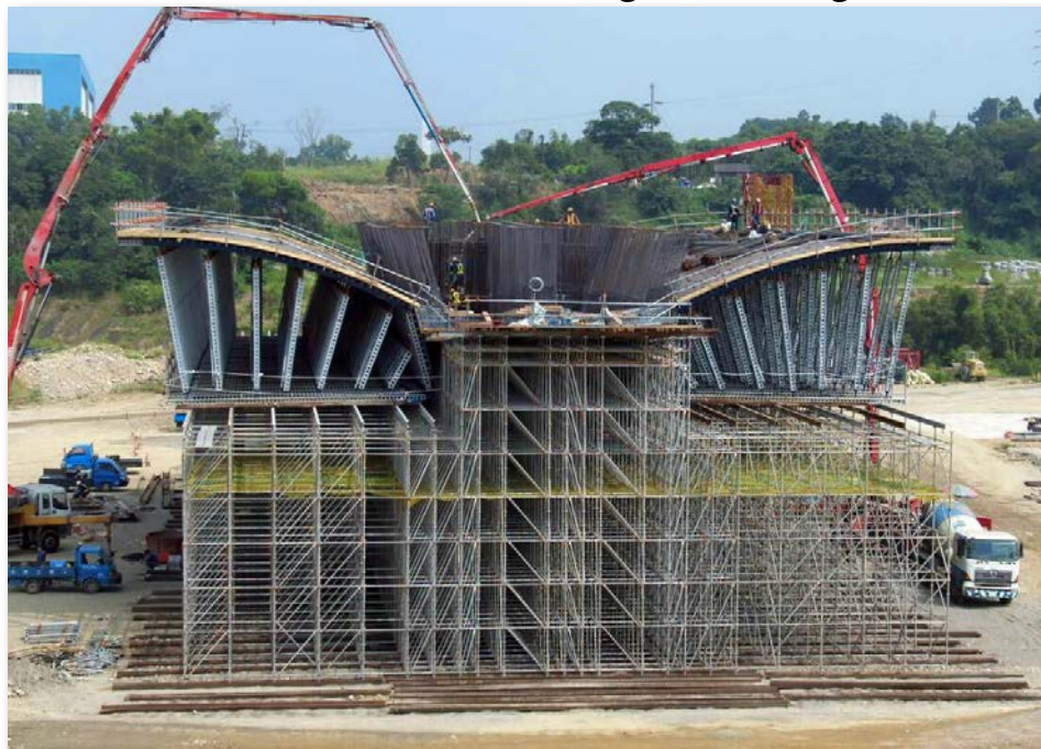
Central Taiwan Science Park - Frontage Road Bridge Formwork
