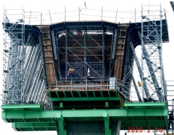
Ankeng Light Rail - Single-Sided Wall 1st Storey
