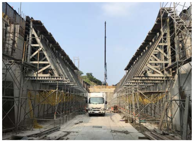
Ankeng Light Rail - Single-Sided Wall 2nd Storey
