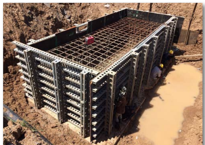
Pier Column System Formwork
