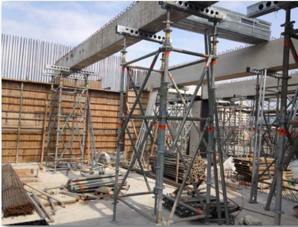
Top Beam as Main Bearer while shoring precast beams
