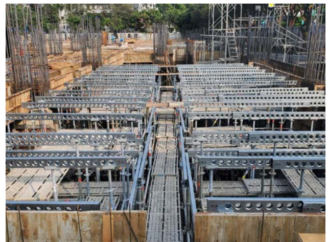
Factory Building - Slab Formwork Top Beam as Main Bearer
