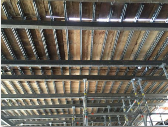
Top Beam connected with H-Beam as Second Bearer on a slab formwork project
