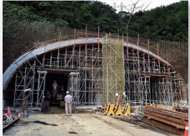
Taiwan Tunnel Arch Form Shoring
