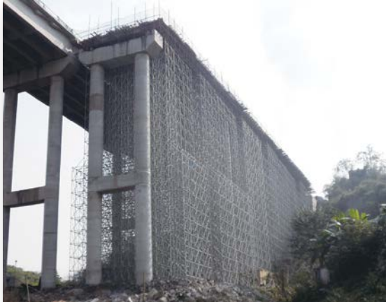
China Chongqing Bridge Three-span Shoring(6-30m height)
