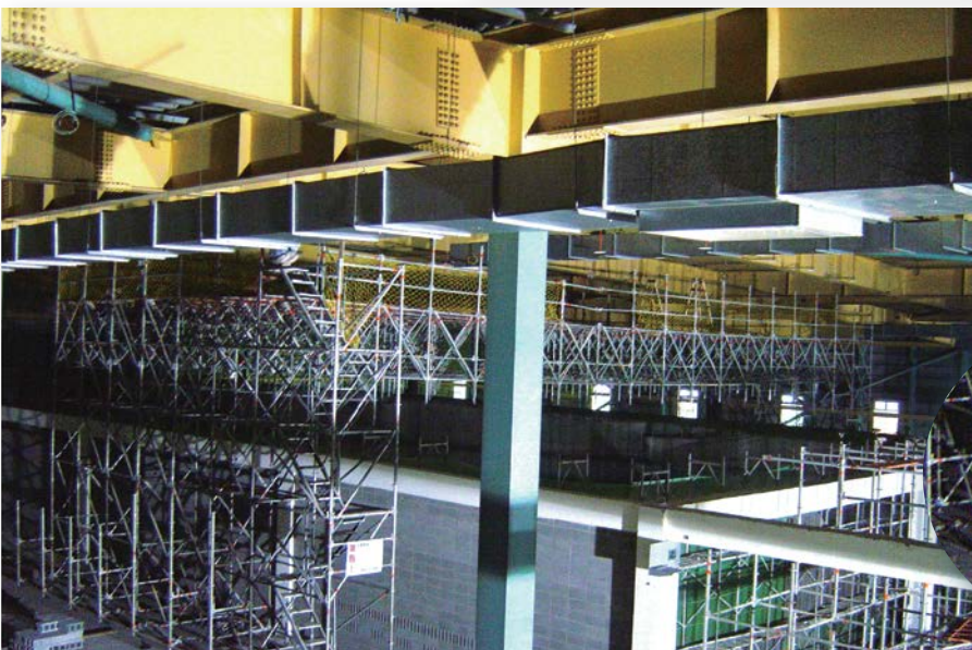
Access Scaffolding for High Level Installation Work
