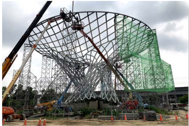
Thailand MRT Station – Shoring for Precast Beam
