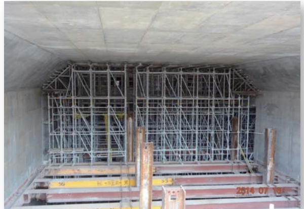
Underground, Cut-and-cover Tunnel Slab Shoring
