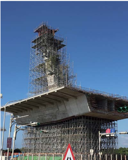
Cable-stayed Pylon - Pier Table Shoring
