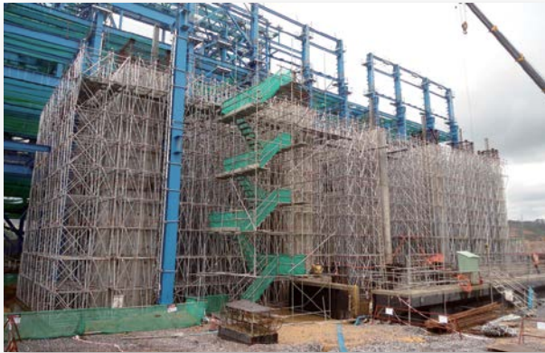
Taipei MRT- Superstructure Formwork and Shoring
