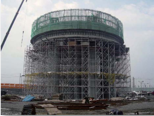
Industrial Park- 3000 tons Water Tower
