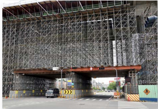
Taichung Expressway No.2 Shoring
