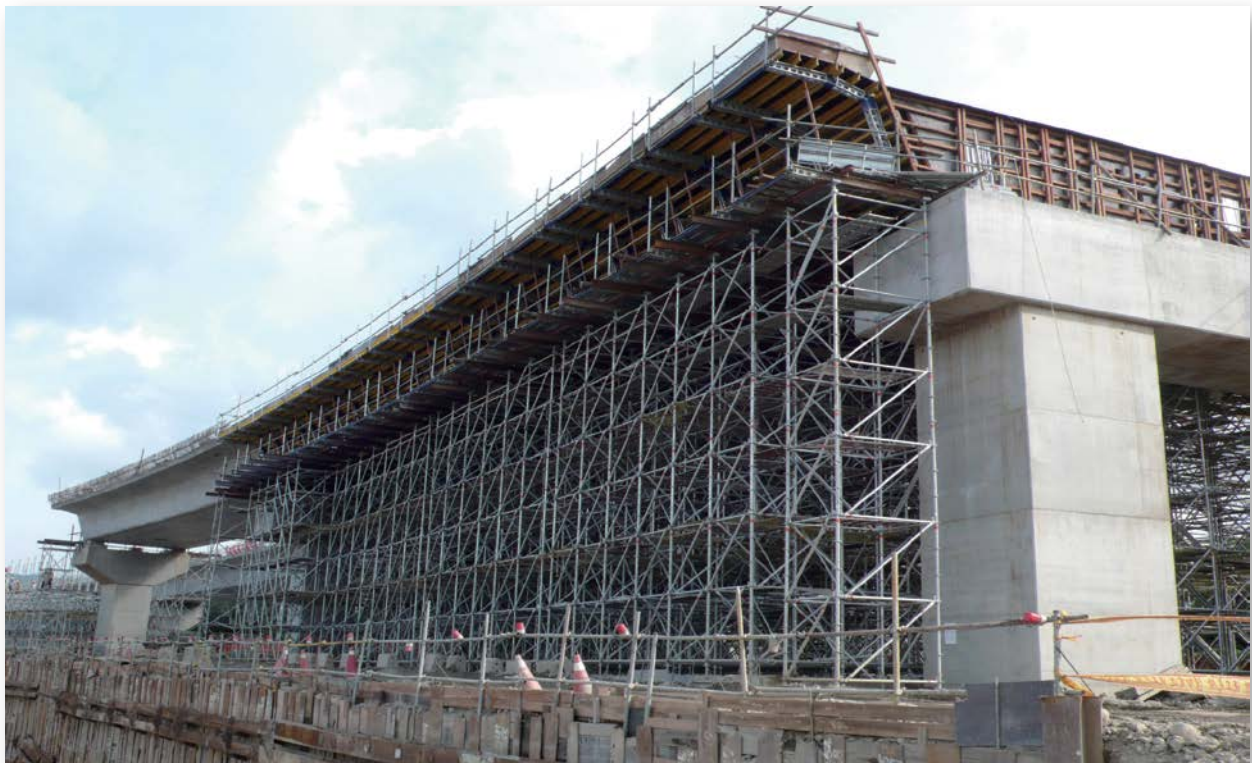
Taipei MRT- Superstructure Formwork and Shoring
