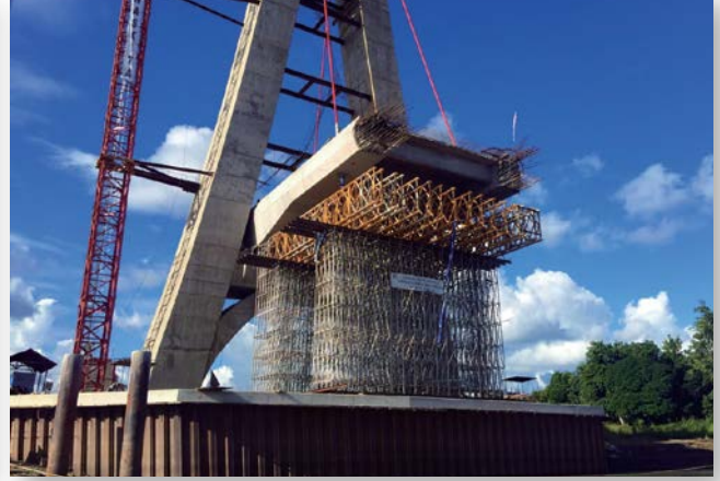
Indonesia Bridge Pylon Shoring
