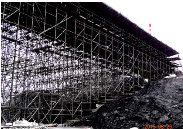
Superstructure Shoring in Slope
