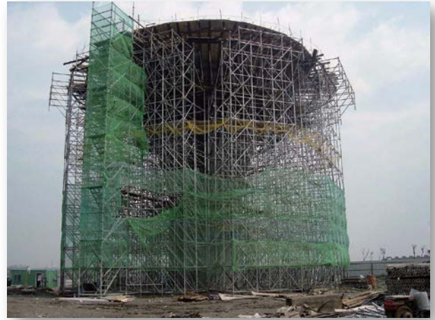
Industrial Park- 500 tons Water Tower
