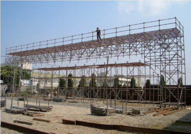
Suspended Scaffolding- Tower and Bridge
