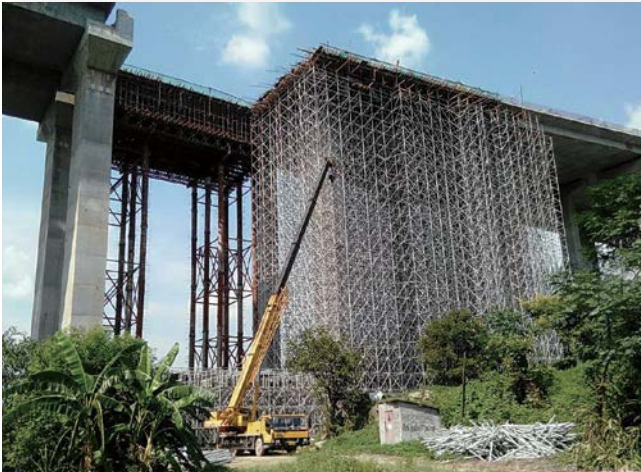
Chongqing, China H:37m Bridge Shoring
