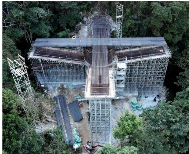
Taipower Tower Base Cross Beam Shoring
