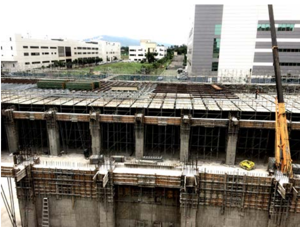
Hi-Tech Factory Slab Shoring
