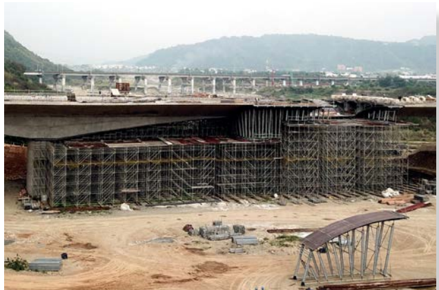
Central Taiwan Science Park Southbound Access Road – Superstructure Formwork and Shoring
