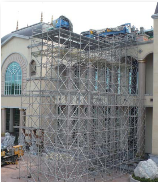
Shoring Platform for Roof Forming Machine
