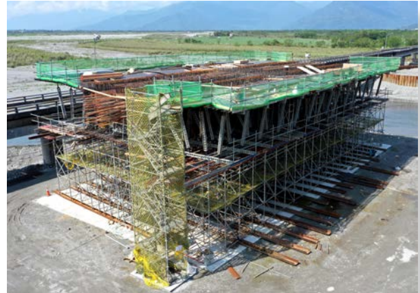
Hualien Jian-ying Bridge Pier Table Shoring
