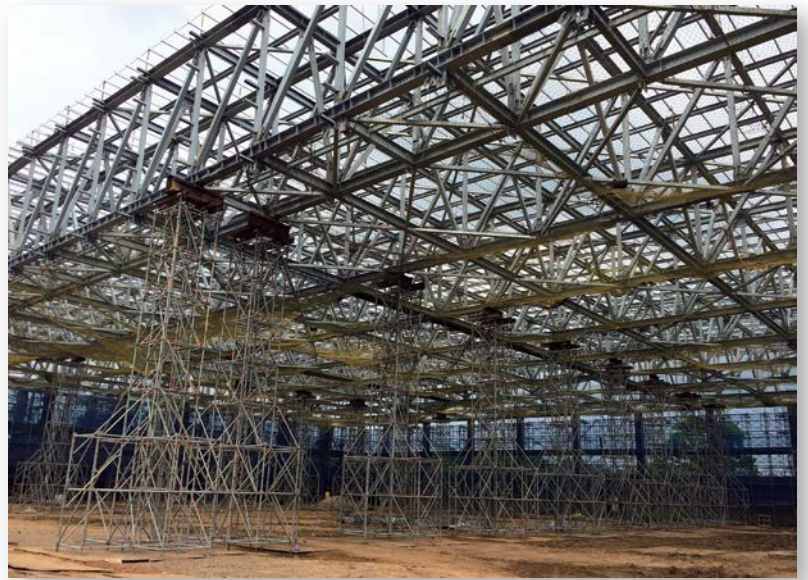
Shoring for Steel Structure Factory Assembly
