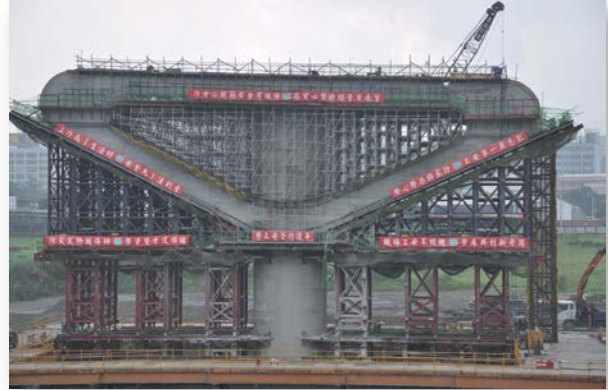
Taipei MRT- Superstructure Formwork and Shoring
