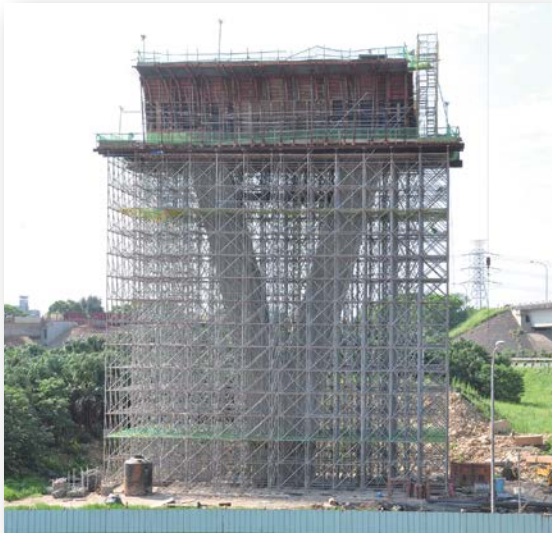
Y-Shaped Pier Cap Shoring
