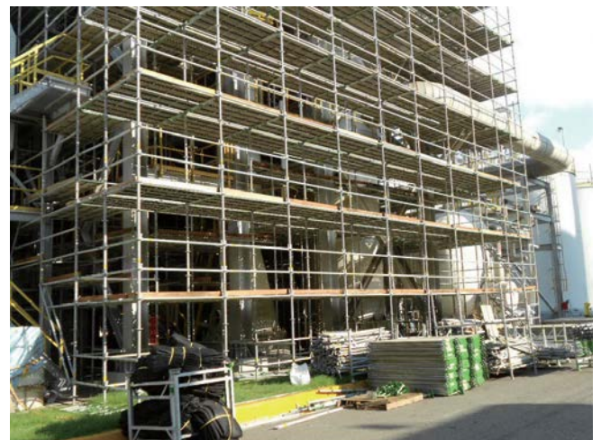
Petrifaction Pipe Annual Maintenance
