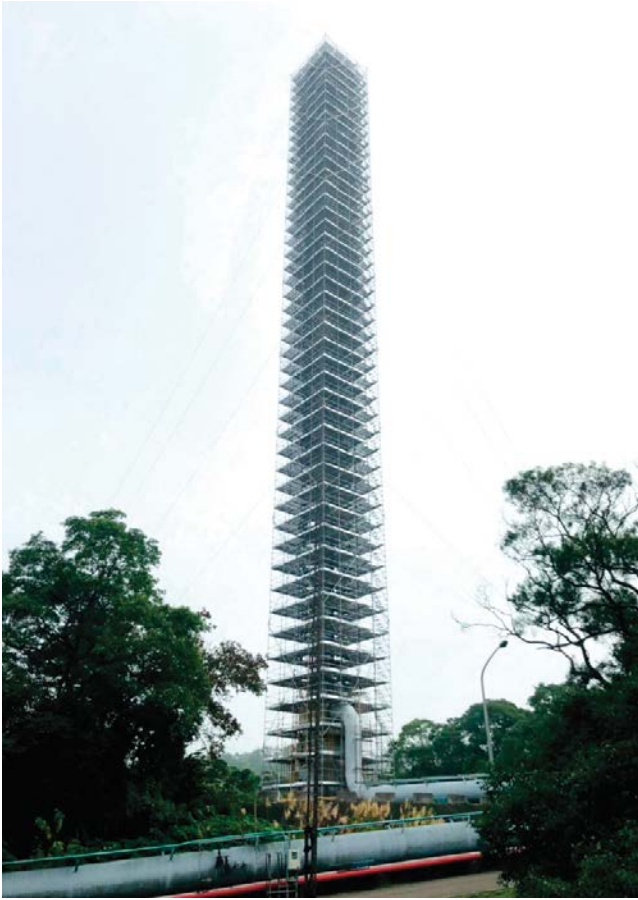
Burning Tower Project (100m Height)
