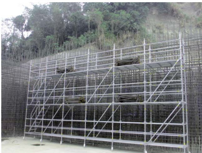
Hushan Distributing Reservoir
