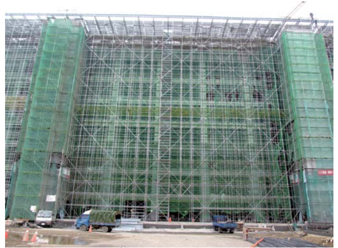
District Court Steel-Structure Roof
