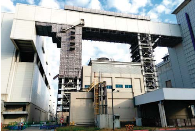
Suspended Scaffolding (36m Height)
