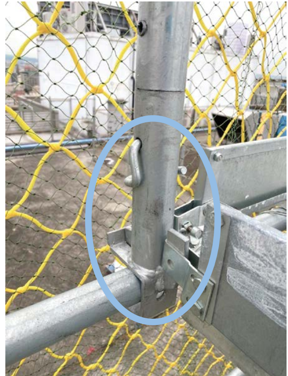
At the staircase corner
