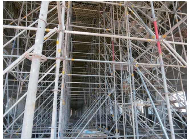
Slab Shoring for Power Station
