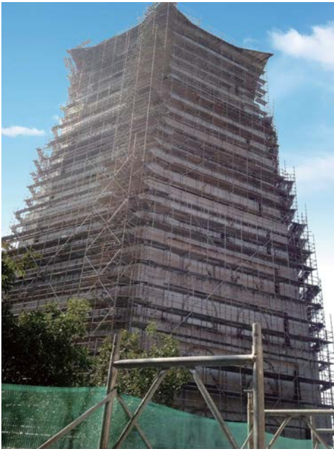
Columbarium Pagoda Refurbishment
