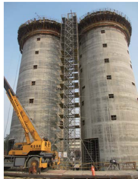
Staircase for Slip Form
