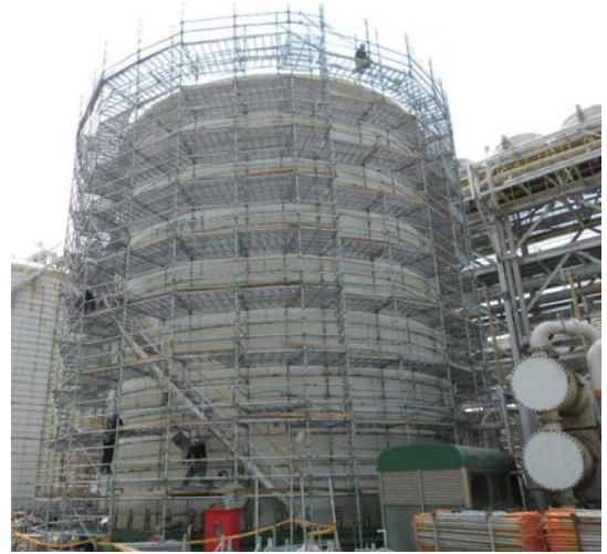
Round Tank Refurbishment
